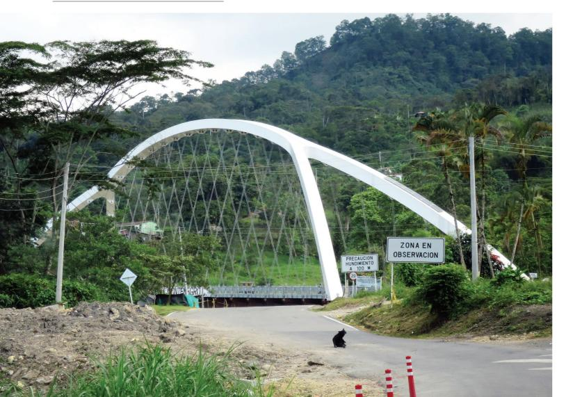
instability of the ground and absorb vibrations. The arch was assembled on the ground with the help of temporary equipment and, once completed, positioned and supported by a system of temporary cables that, hooked to a
