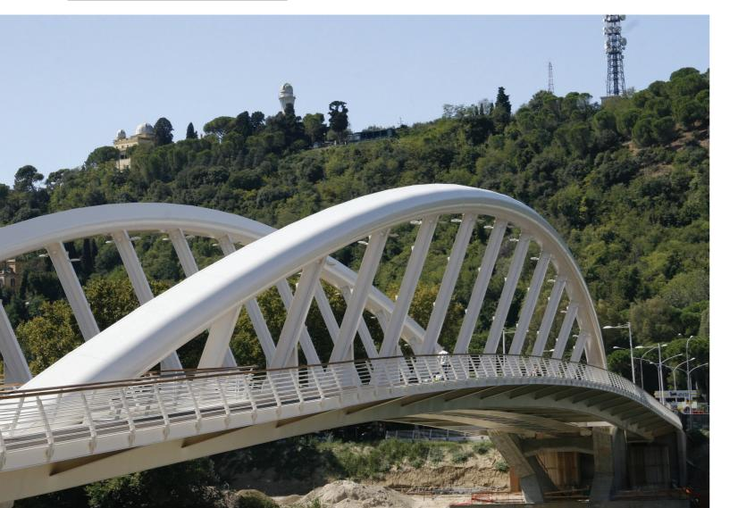
a height of 30 meters. After installation, the two diverging arches have been fixed on one side and left free to slide on bearing on the other. The peculiarity of the structure is the presence of six steel cables inside the deck supporting its weight: only when these cables were properly tensioned,
