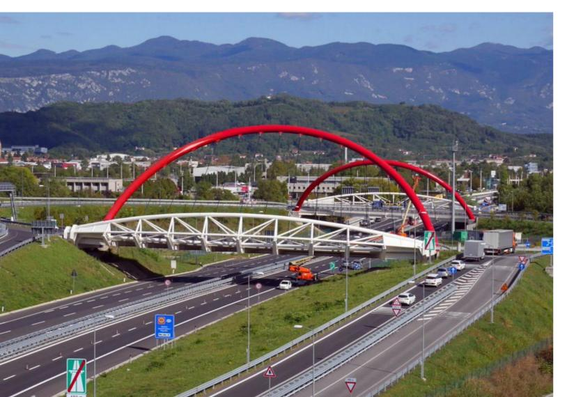
main phases: they were first raised horizontally by using a 300-tons crane and then, with a slow rotation, raised and turned. Finally, two 120-tons cranes placed on the side
