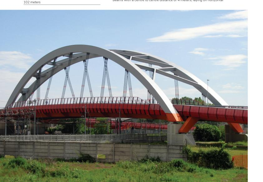
double-T elements 2 meters high. Altogether, the structure has a weight of 1.700 tons. The assembly phase took place without interfering with the below railway traffic: firstly it has been pre-assembled on the ground with the aid of
